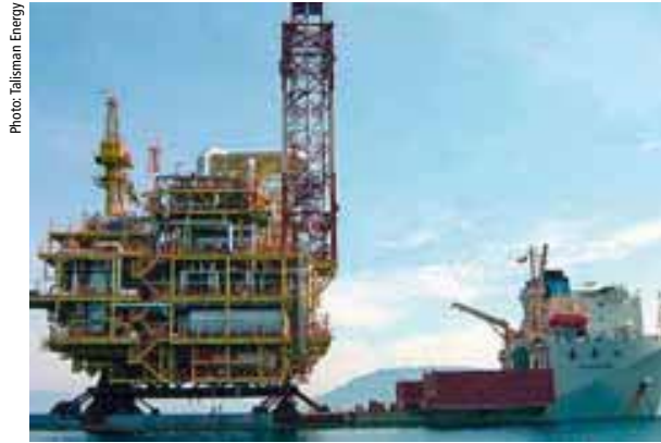
TRANSPORT. A Talisman topside being transported to its destination, the PM-3 project between Malaysia and Vietnam.
